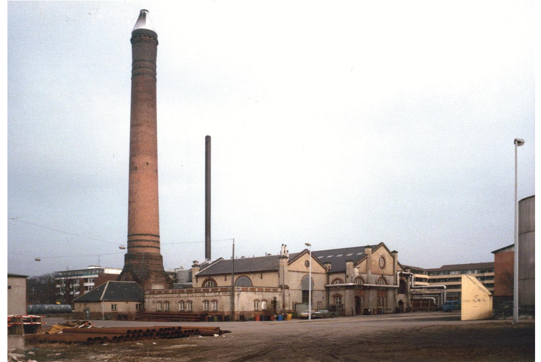
Picture: Frederiksberg Utility, the first district heating plant in Denmark.
