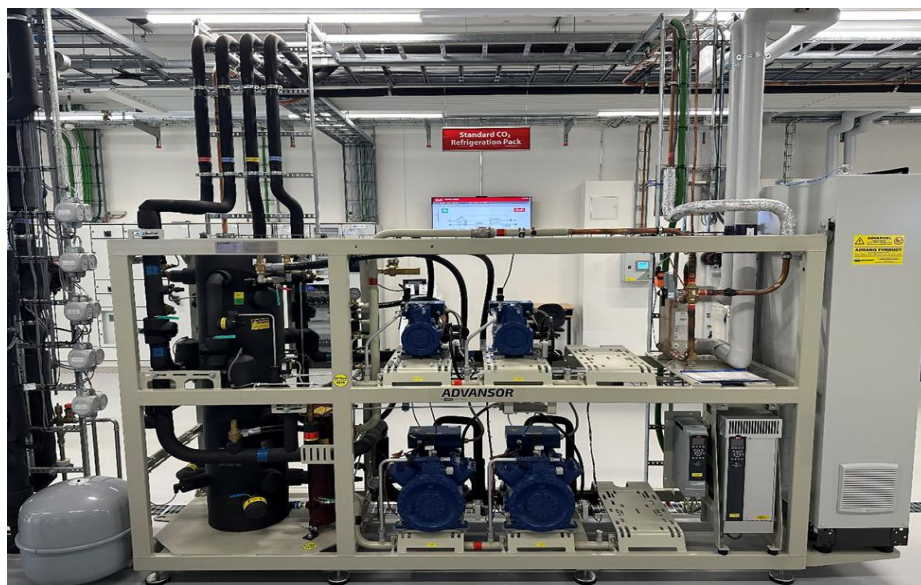
Fig. 4.4. CO 2 refrigeration machine in supermarket
