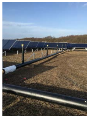
Fig. 8 and 9 - Standpipes made indoor. In the indoor factory straight pipelines are manufactured with standpipes, designed so they match the exact position of the solar panels.
