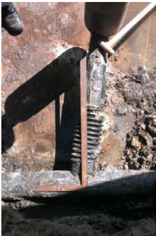
Fig. 1 - Branch, damaged by large movements.
