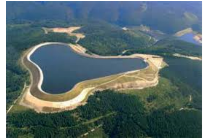
Pit heat storage up to 1.5 – 2.0 mio m 3
