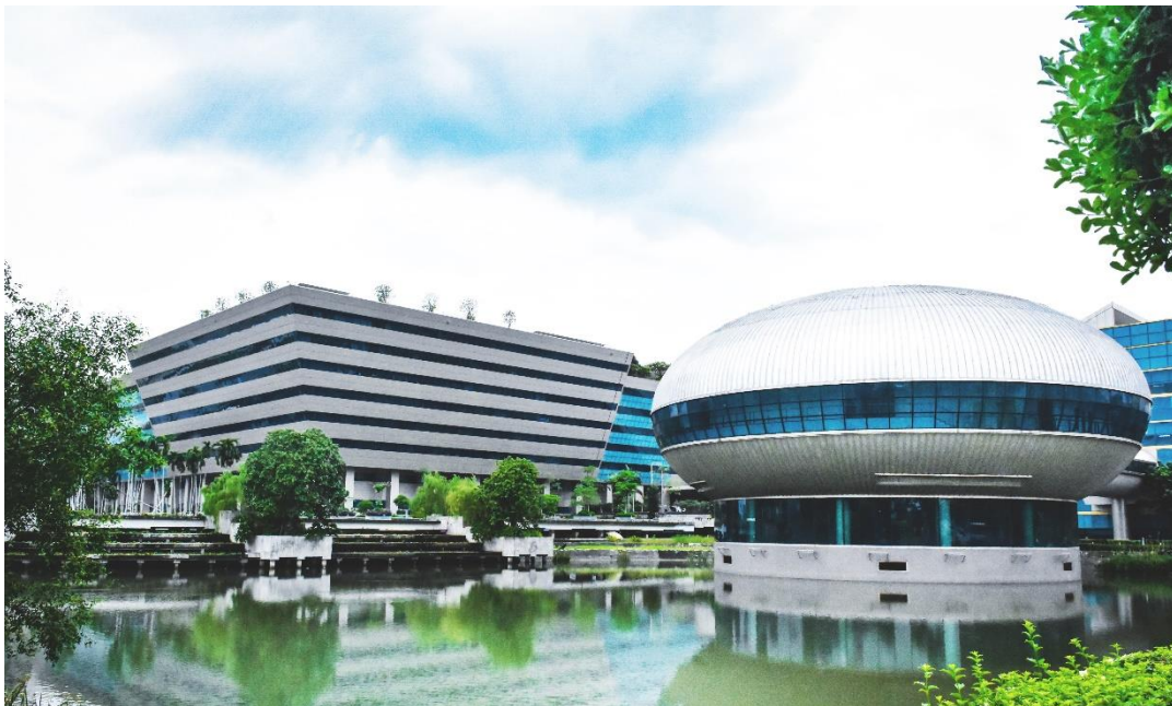
Figure 8 Cooling Pond around The Main Building (BM)
