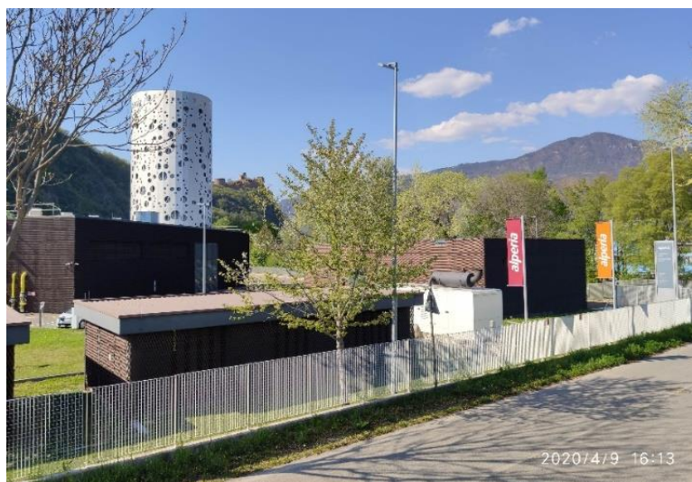
image 6: sight of the complete DH plant with pump station in the front and the thermal storage tank in the background (source: Alperia Ecoplus)
