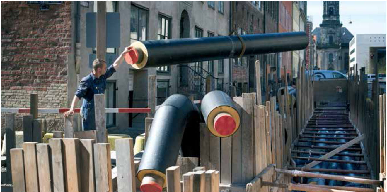
Figure 10: Installing new DH pipes in Copenhagen
