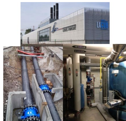
Figure 31: Chartrons DHC: WWTP, non-insulated pipes and substations (source: EDB)
