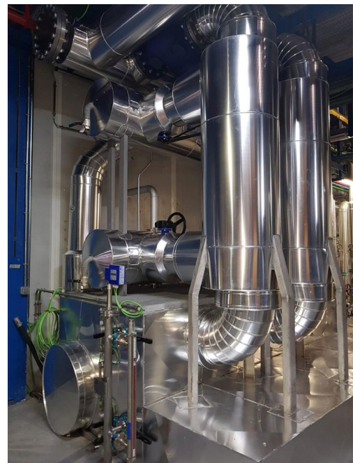
Figure 49 : Waste heat exchanger (steam/water) at the tyre manufacturer plant (source: REBI)
