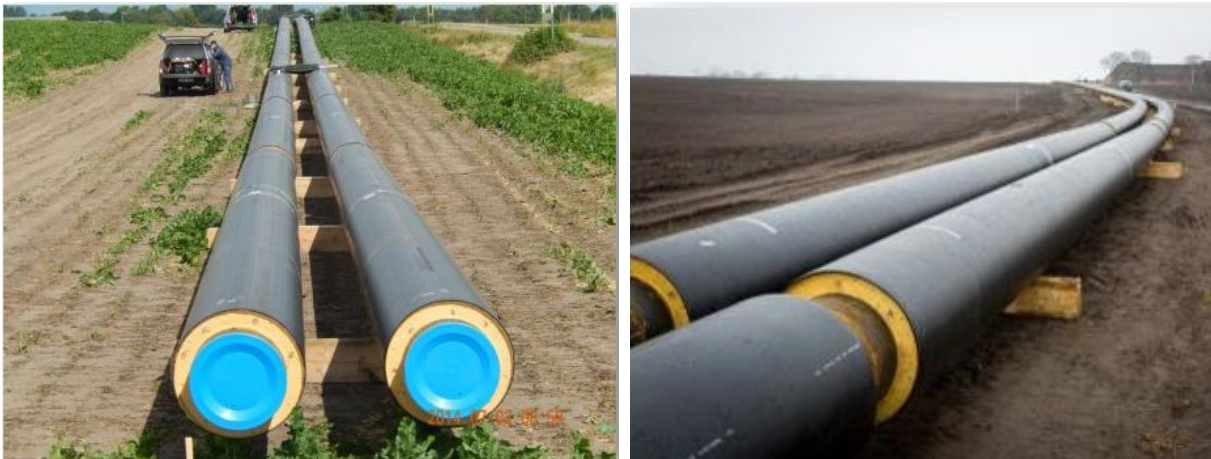
Figure 26: Evita interconnector DN500 pipes (pictures from the construction works by Mr Jan Lindeberg)
