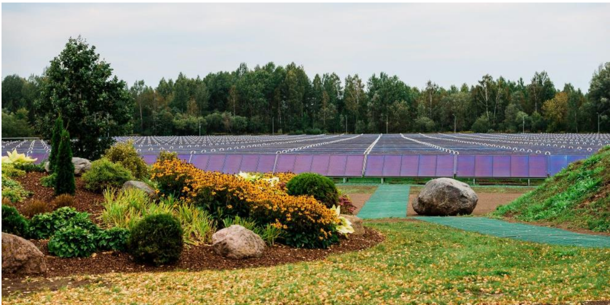
Figure 7. Solar collector field for network Salaspils (Bankwatch, 2019/Photo by Kaspars Suskevics, CC-BY-NC-ND)
